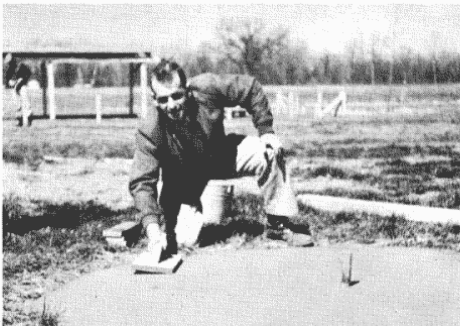
Concrete for center of carrier deck circle is finished off by Charles Eschmann, head of Greater St. Louis Modelers Association. A real working prexy!
