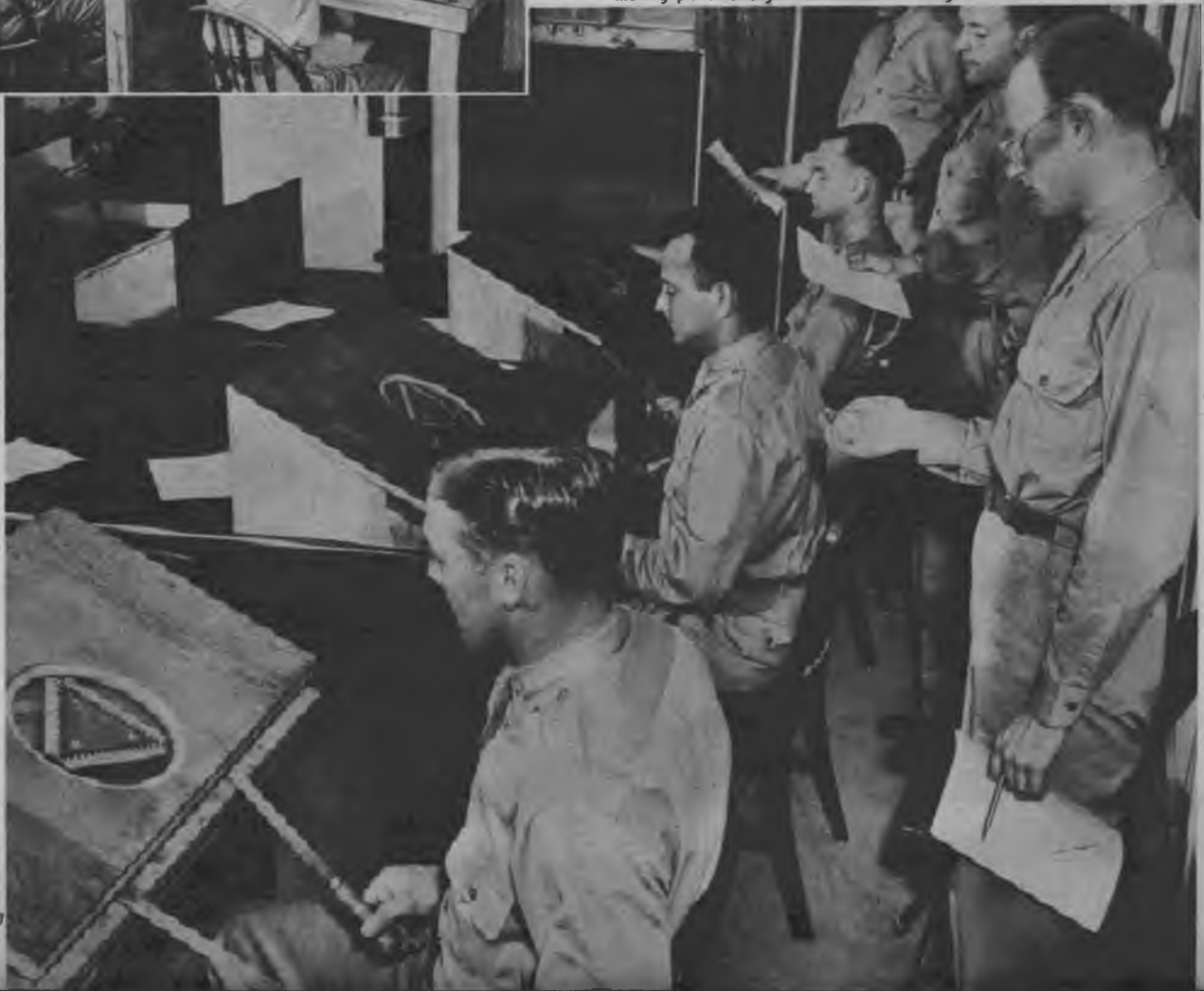
In this test, co-ordination between both hands of student is measured by moving pin in straight line around a triangular course with the two levers.
