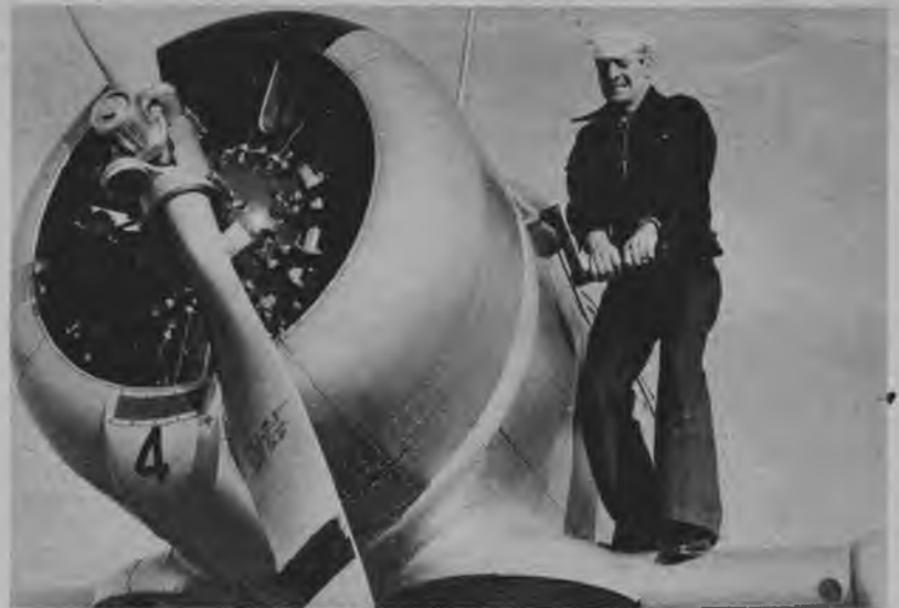
He both flies with them and keeps them flying. Here he cranks inertia starter on SNJ.
