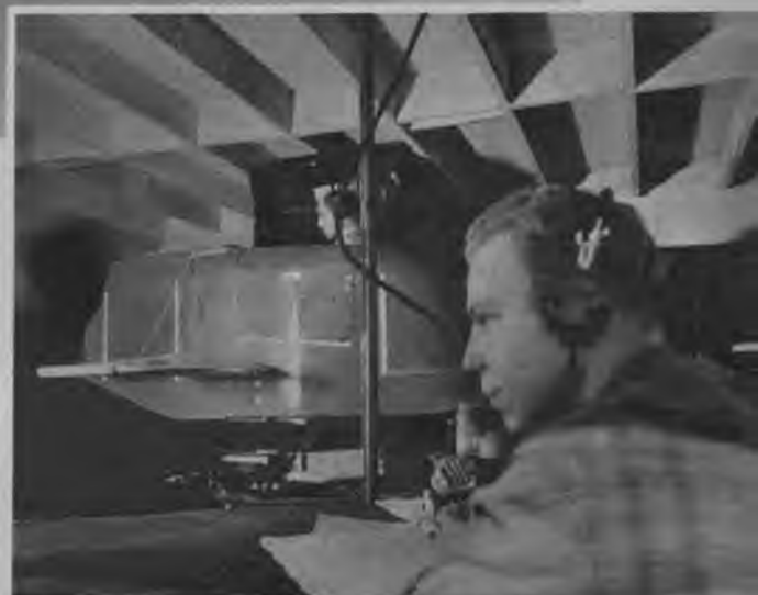
Before doing any actual night flying, the student is taught the rudiments of instrument technique on this Link trainer.
