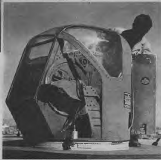
Closeup of Consolidated tail turret, sans twin .50-caliber guns which have effective range of 600 yards.
