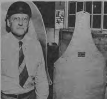
Two types of armor protection. Left, "booth" for bomber pilot and, right, plate armor for pursuit seat.
