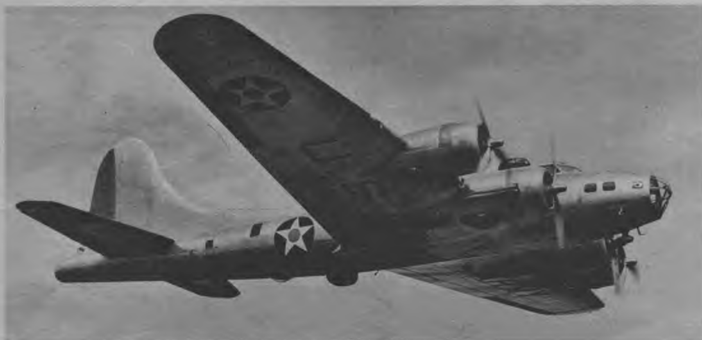
This striking flight photo of the new Boeing B-17E Fortress shows the many new features of this sensational performer of the stratosphere. This new heavy-duty long range bomber has added fin area for directional stability in making bombing runs in the thin air of high altitudes, new tail, top, and belly turrets and nose-gun positions
