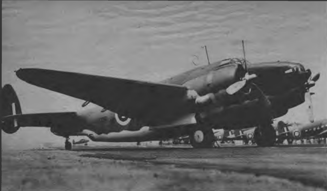
The Lockheed Ventura, developed from the popular Hudson bomber, features more power (nearly 275 m. p. h.) and a rear belly turret the Hudson lacked.
