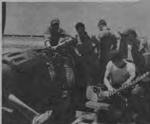
Joined by metal links, the cannon shells are fed into the removable magazine box.
