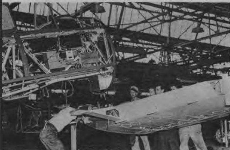
The body grows wings. Here the wing section complete, with the exception of outer panels, is added to the plane's fuselage. This inboard wing section will contain the landing gear.
