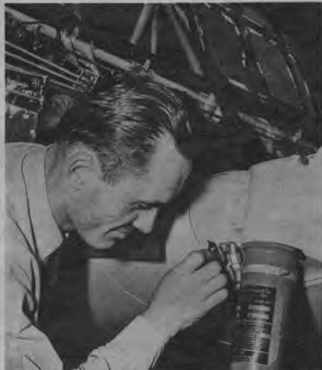
Final company O. K. is applied after rigid inspection. Here hydraulic line to brake is approved. Later, army inspectors also give ship a complete check.
