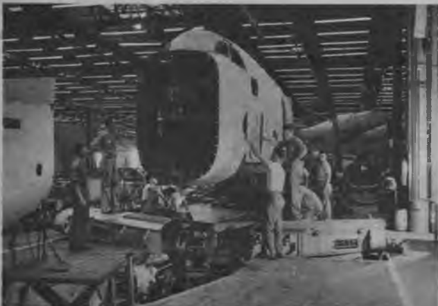
Here a Ventura fuselage is being guided into place in the mating jig where the wing center section will be attached. The Ventura is the army's B-34.
