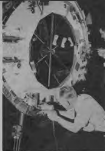
Wheel of fortune. Here a rib for B-26 is formed on a wheel fixture that permits men to work at any elevation.
