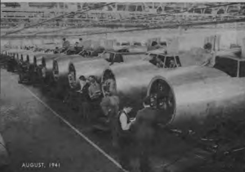
Mass production. A line of B-26 noses moves toward final assembly. This gives some idea of quantity of bomber production. The trick in mass production of airplanes is to complete smaller assemblies as far as possible before bringing them together.
