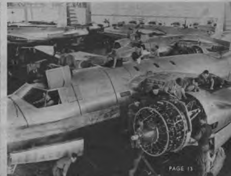
Swarm of workers put the finishing touches on a flock of B-26s on final assembly floor. Here are installed 2,000 h. p. Pratt & Whitney Double Wasp air-cooled engines. Martin B-26 was one of first American types bought off the drawing board.
