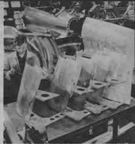
Sub-assembly. Hundreds of such operations form 25,000 parts into sub-assemblies which ultimately come together as finished B-26.
