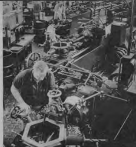
Worth their weight in gold, these highly flexible machine tools in the Martin shops machine castings and forgings to the thousandth of an inch.
