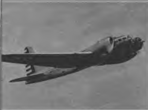
Twin-engine medium bomber by Douglas. B-23 with tail turret is an improved version of the Douglas B-18A.
