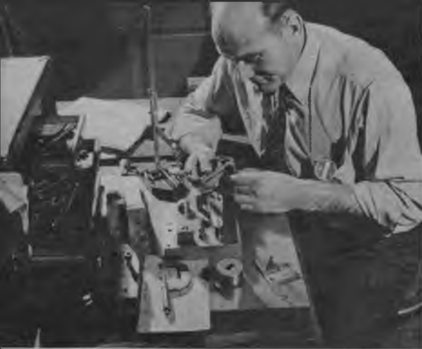
Toolmaker's craft is one of oldest in the industry. This expert is measuring to extreme tolerances a tool intended for a Martin bomber. Skilled toolmakers are much in demand.
