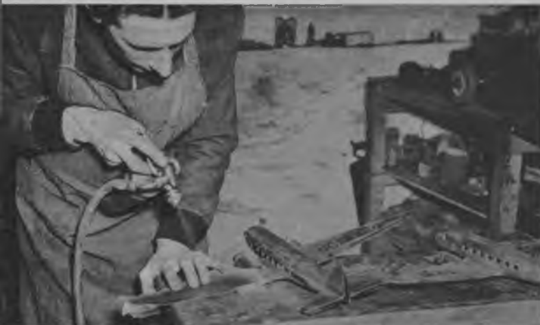
Paint trimming is done with an airbrush. The unpainted sections are protected by metal mask. These models are seen on display all over the country in air transportation offices.
