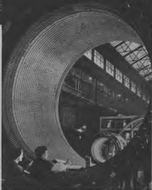
Power to blow away. This is stationary part of the 40,000 h.p. fan motor to drive the propellers at Wright Field tunnel.
