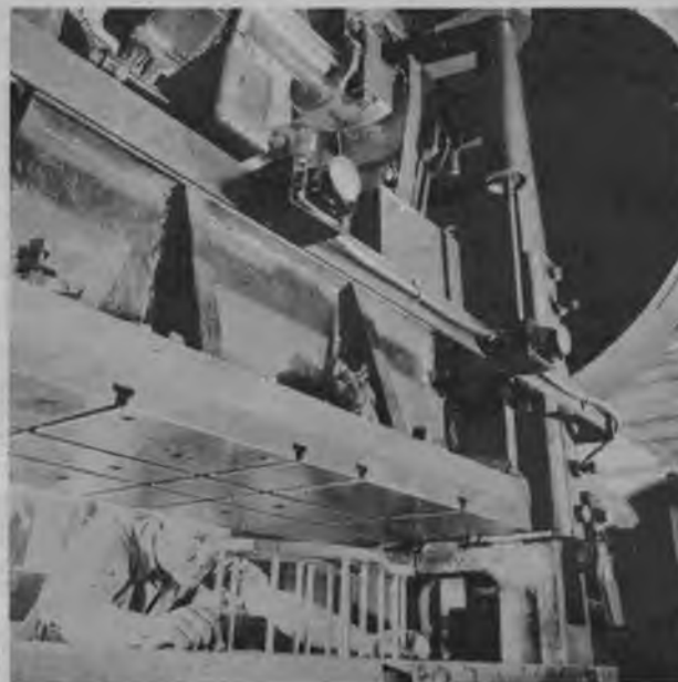
Punch press. One of a battery of powerful presses which form out metal parts rapidly. An operator sets a die for the job. Acres of machines of every description work right around the clock at Martin.
