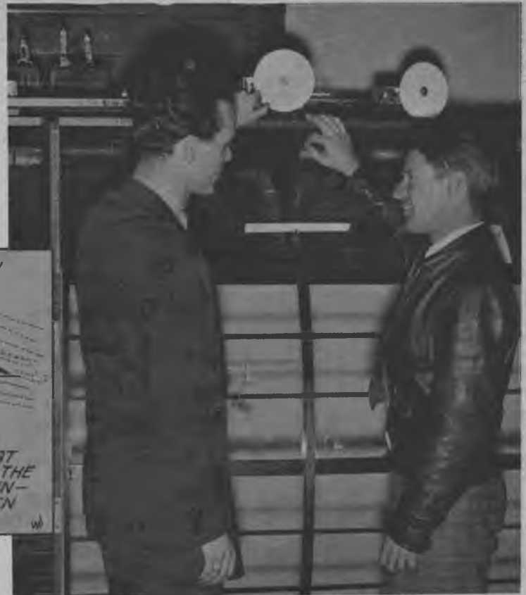
Bill Tyler, left, shows Doug Corrigan details of the Jordan-Marsh slow-speed model wind tunnel in Boston. Model aerodynamics are a specialized problem.
