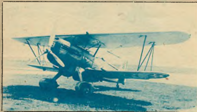
● The XP-6H was first production P-6E with four extra .30 cal. machine guns installed in wings. P-6E started out as XP-22, which was development of P-6A with entirely new nose and single strut landing gear. Became most famous of Hawk series.
