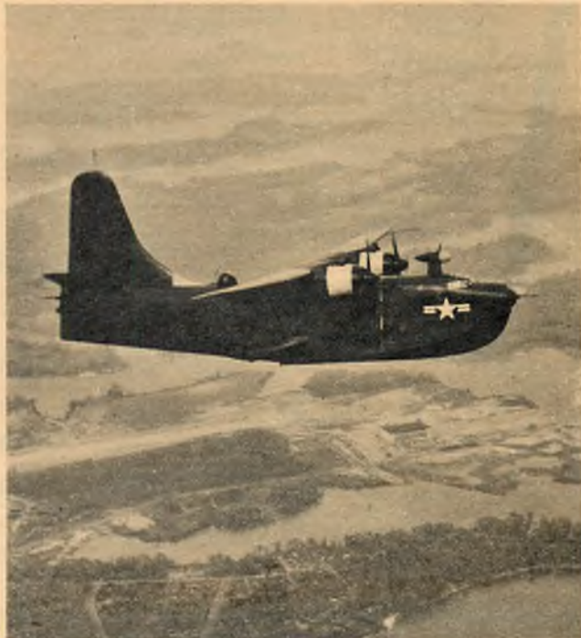
● Navy's experimental patrol boat Martin XP5M-1 features long after-body hull for landing and take-off in rougher sea.
