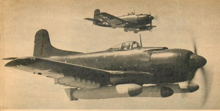
• A variety of armament can be carried by the AM-1. Lower plane has three torpedoes, six bombs; upper, a 2000-lb. bomb, 14 rockets.
