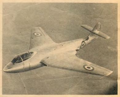
• British experimental jet fighter the Hawker P.1052, is the development of the earlier P.1040. Powered by the latest Rolls Royce Nene engine developing over 5,000 lbs. thrust. Plane has double entry wing root air intakes and double exhaust nozzles.
