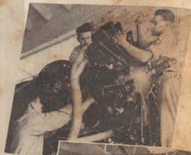
Power plant installation
