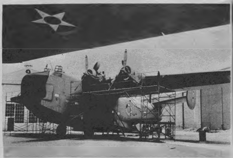
Outdoor check. The huge Consolidated PB2Y-2 flying boats are given their final check inspection outside the plant to make room for those coming along behind.
