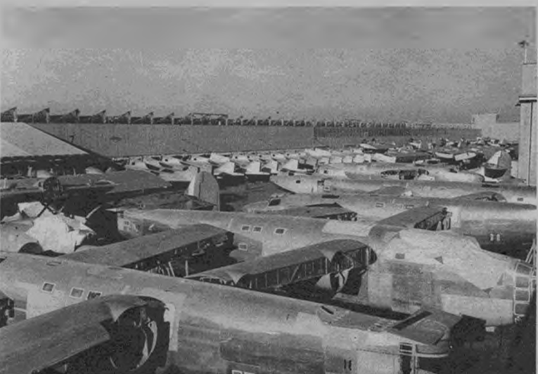
Output builds up. The partially finished B-24's and PB4Y's fill every available inch of space about the huge factory yard. Note the tail turret location at the lower right.
