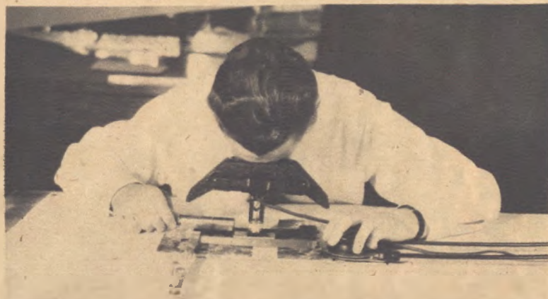
● Stereoscopic viewing devices are a big help in certain types of mapping work. Only with their aid can surface elevations be correctly established.
