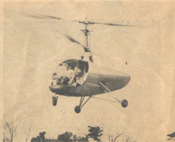
● The Commuter, produced by Stanley Hiller, Jr., is a compact helicopter featuring unified control system.
