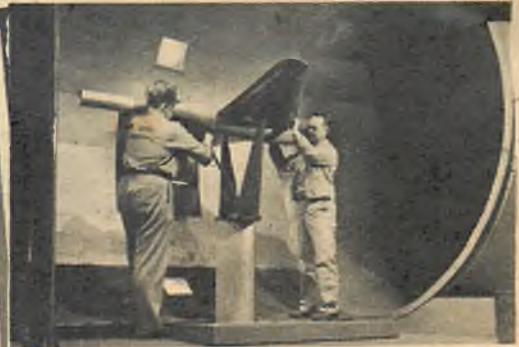
Aeronautical Engineering offers you a wide choice of creative and practical duties. Here two engineers install a guided missile model in the Northrop Aircraft, Inc. wind tunnel to study its aerodynamic characteristics.
