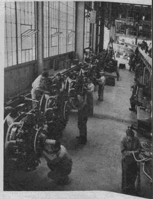
Engine assembly line. Here the wiring and exhaust units of the power plants are attached and checked.
