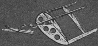
Simplified turned-up wing tip construction by Vermoch.
