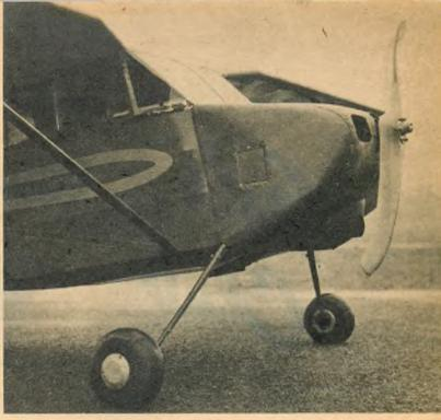
Steve Wittman, famous racing pilot, designed this lightplane, the "Buttercup." Top speed 130 mph. It lands at 30 mph. Gear flexes fore and aft. Even the prop was designed—and built—by Steve!
