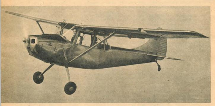
Cessna L-19A, latest liaison plane for Army field forces and National Guard. Powered by a Continental 0-470-11 of 190 hp.
