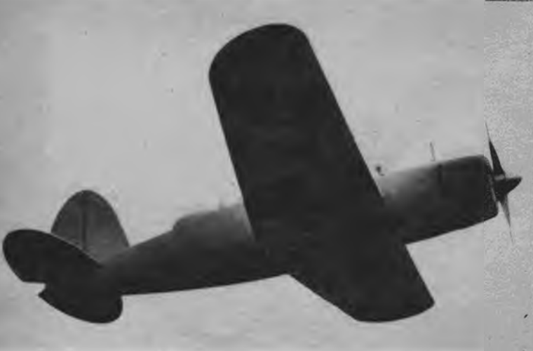
Newest dive bomber. This Brewster Bermuda carries 1,000-lb. bomb within fuselage. Has twice range of German types, powered turret.
