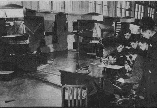
Blind-flying training at Kelly Field is done with this battery of Link trainers. Mechanical "crab," foreground, traces the pilot's course.
