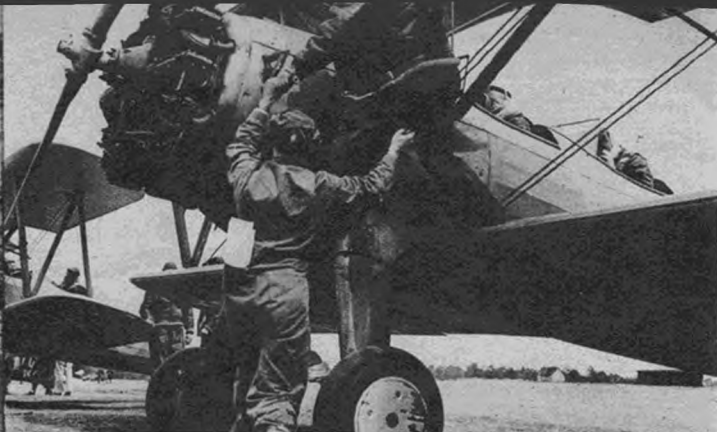
250 h. p. Continental engine of this Stearman primary trainer is started by cranking inertia starter. Small flywheel stores energy to kick over engine.
