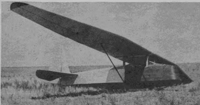
All-wood wagon. This home-built sailplane is modeled after the Prueffling with a special wing. Harland Ross flew it to an altitude of 7,000 feet.
