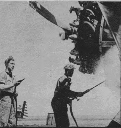
Don't be alarmed. It's not a fire. Pressurized soapy steam cleans grease and oil.
