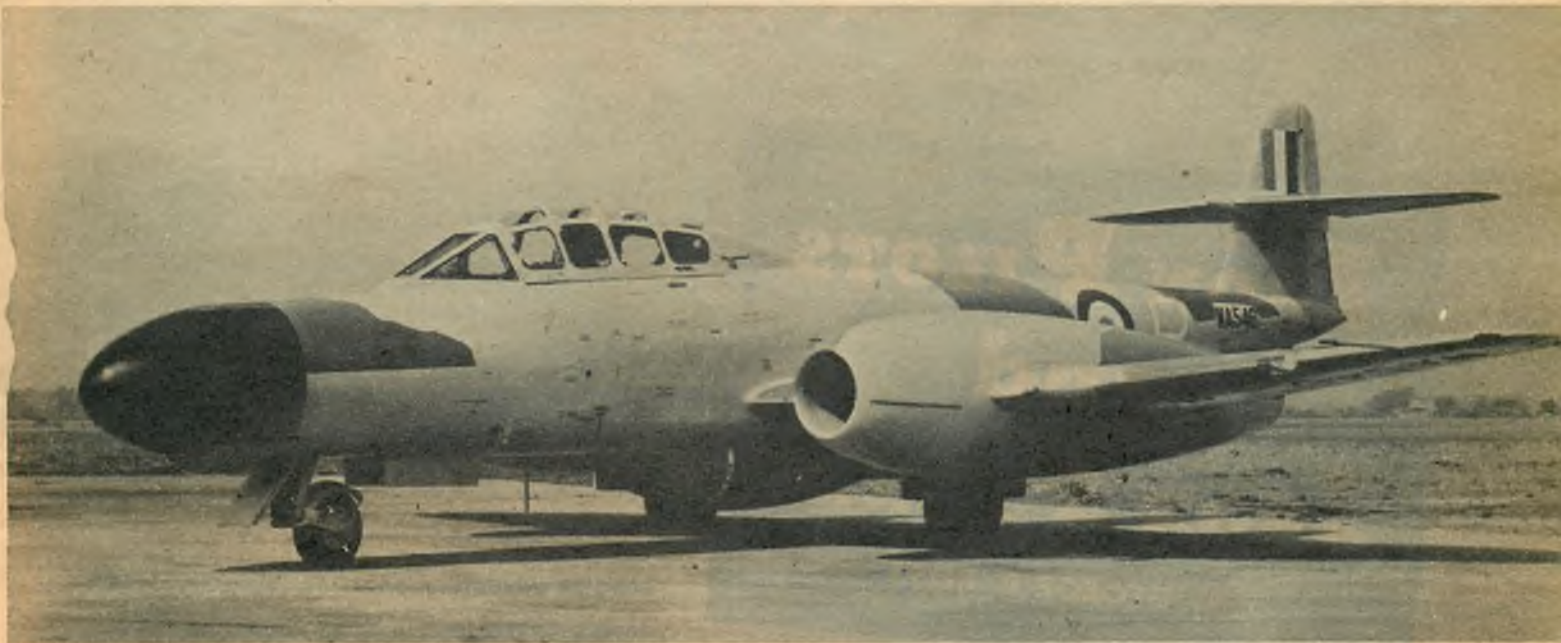
Jet night fighter. British Gloster Meteor NF.11 adapted from standard fighter for night duty. Plane has large radome in the nose,
