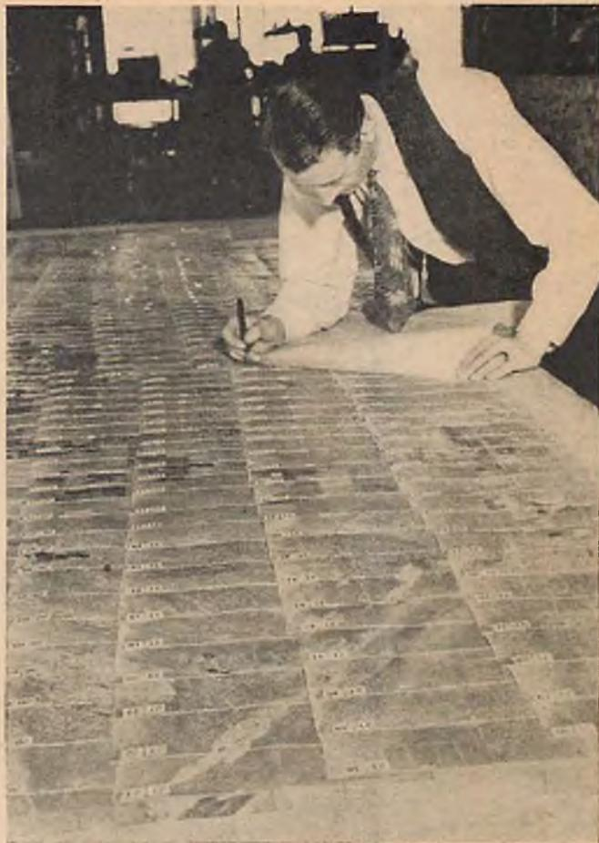
**Two**—These photos are carefully numbered and placed with millimeter precision upon a huge drafting board scaled with latitude and longitude lines. Skilled cartographers cut and fit the photos until the whole area is fitted like a jigsaw-puzzle.
