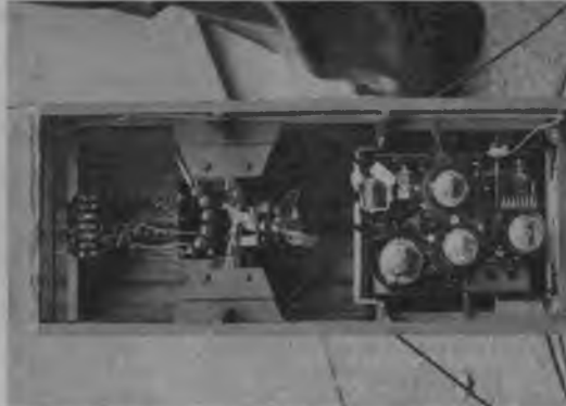
Left—This successful model was built by Joe Raspante, of Brooklyn, N. Y., here shown testing four-tube receiving set. Heavy-duty batteries are used for testing to preserve the plane's own, smaller batteries.
