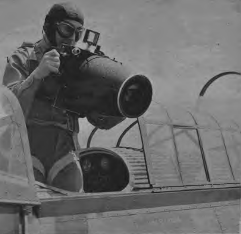
Photographer with camera for vertical or oblique work. Camera takes 110 7x9 shots on 75-ft. film.
