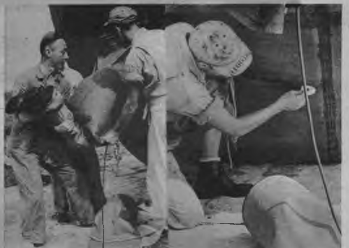
Left above—Curiosity killed a cat. Supervisor crawls into balloon to look for leaks. Right—A rigger marks leak with chalk for subsequent patching.
