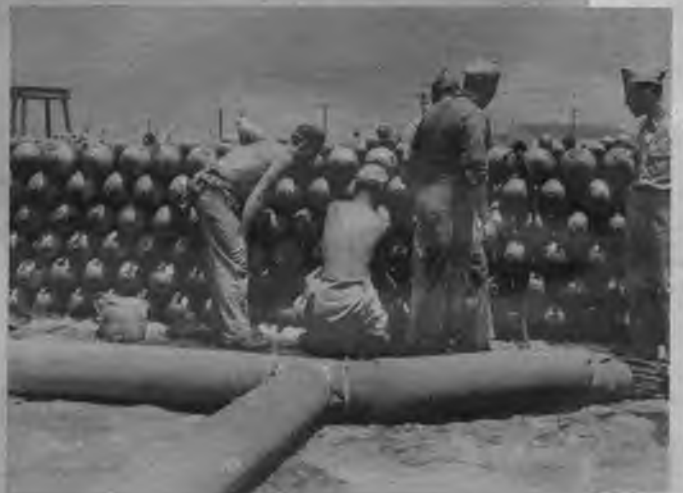
20,000 cubic feet of helium is fed into each barrage balloon from 150 of these gas cylinders. T-shaped pipe in foreground leads to the balloon.
