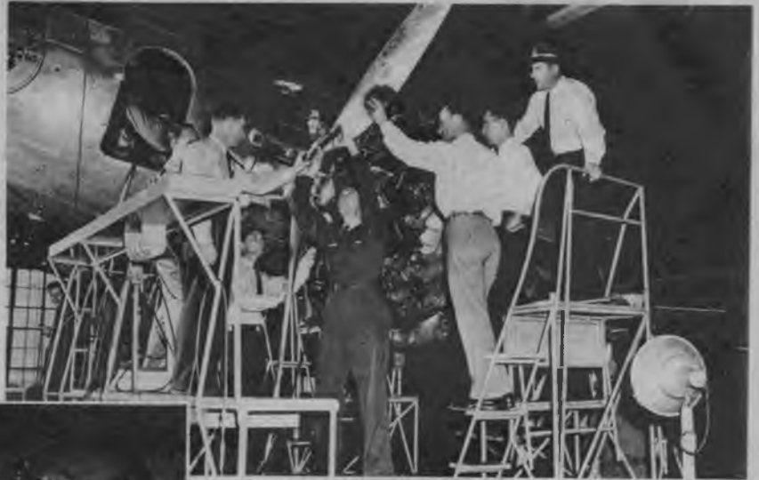
Lots of work ahead. Post-war expansion in air freight and passenger carrying will call for more trained maintenance men.
