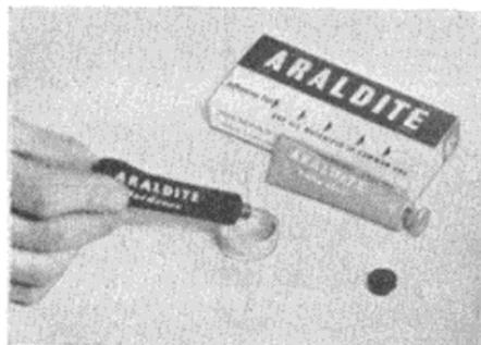
Aero Research have packaged a special form in two tubes—one containing resin and the other
