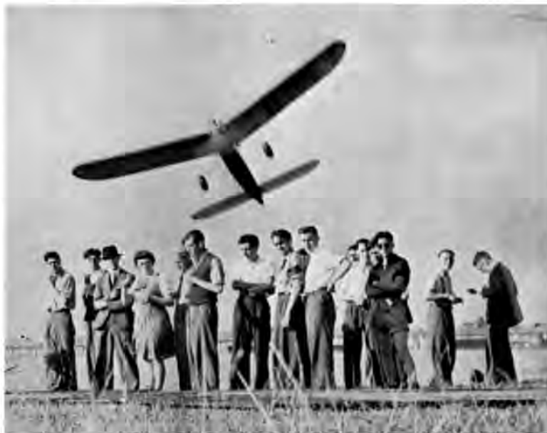
An example of bad take-off. The model has turned violently to the right and is already at right angles to the take-off board.
