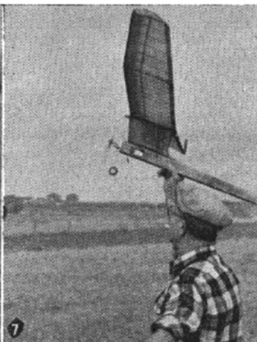
5. Raymond Shirt with his PAA-Load endurance model, the first of its kind in this country. He tried to break the American held record. Model carried 1½ lb. cargo, 8 oz. pilot and 1 pint of fuel. Power was Oliver Tiger converted to rotary disc valve—model used very little fuel in successive attempts totalling 105 minutes.
