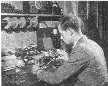
Assembling transmitter chassis in the radio department.
