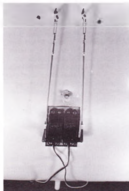
Servoinstallation i vingen
