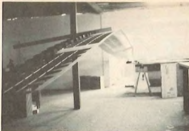
The wing loaded to 5.3 G stress.
