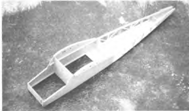
Tail pulled together and bottom partially sheeted.
