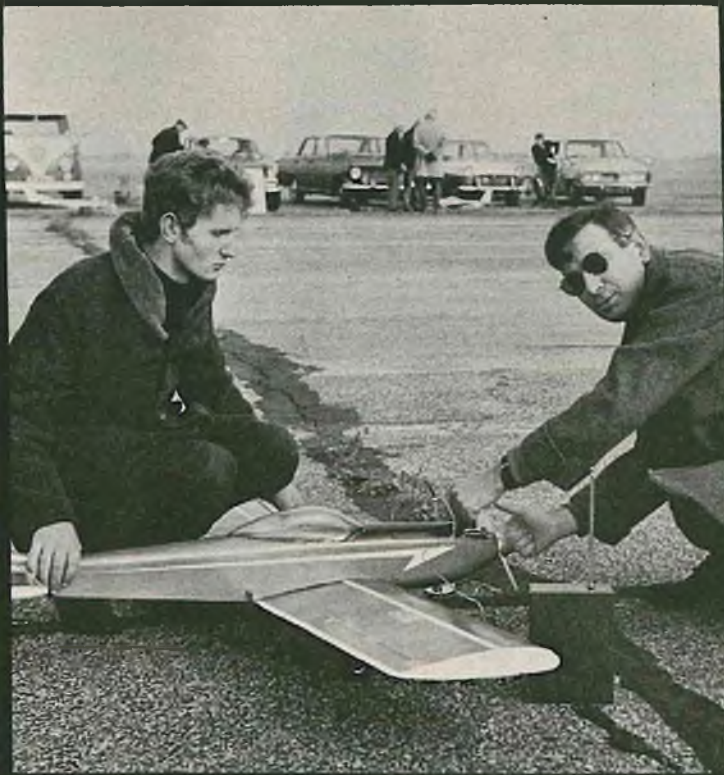
Left: Chris Olsen about to start up for Round #2. New "Uplift" model has parallel chord wing with inset ailerons. Contestant Bradley is acting as Chris's mechanic.
