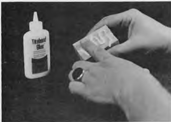
Shear web edges are coated with aliphatic glue, separated and allowed to dry before installation.
