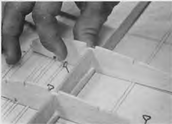
Note proper fit of shear webbing between ribs.
