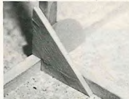
Addition of triangular Lite-Ply gusset ties vertical and cross member together and strengthens the cross section preventing it moving out of square. Fit should be as close as possible for good gluing and for greater strength.
