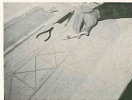
Hypo handy for applying cement in holes.
