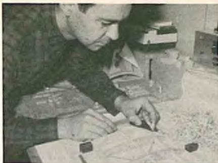
Block plane used to finish wing tip to cross section.
