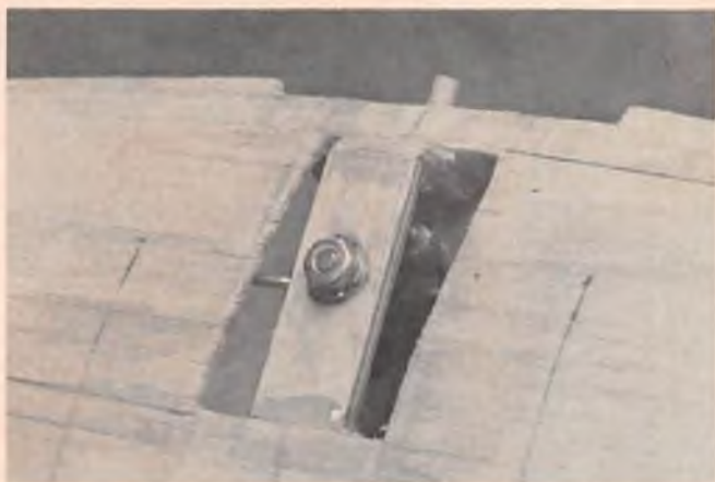
Another view of the servo wheel mount. Position of the actuating rods indicate that the gear is extended.
