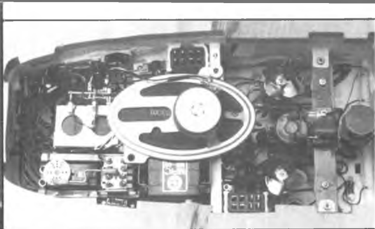
Layout of electronic equipment as viewed from the underside of the deck cabin.
