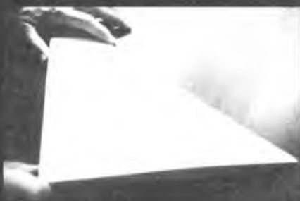
Completed surface, ready for paint.
