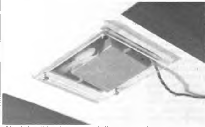
Plastic box lid — 3 screws and silicone adhesive hold it firmly in place.
