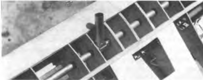
Underside of wing before sheeting; showing tubes fitted into "T".
