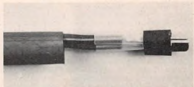
Charger plug installation, shrink tubing over each pin, with a larger piece which will go over the entire plug rear and body.
