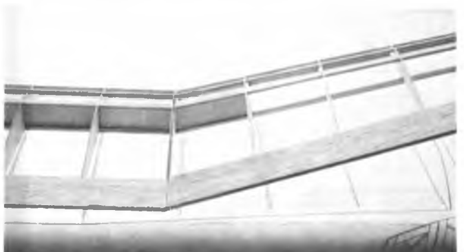
Slide tips on — Zap in place.
