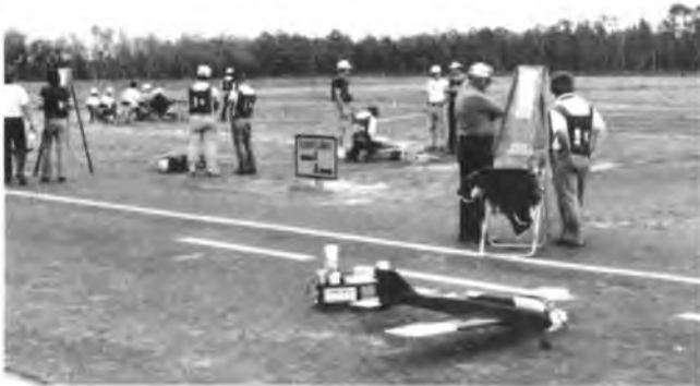
General view showing runway and taxi ways.
