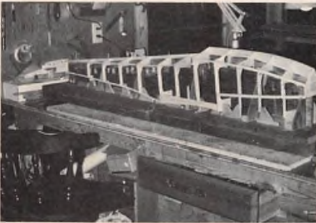
Basic frame work of hull has been completed at this point.
