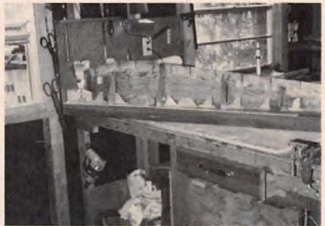
Author's hull jig on work bench. To date, five hulls have been built on this jig.
