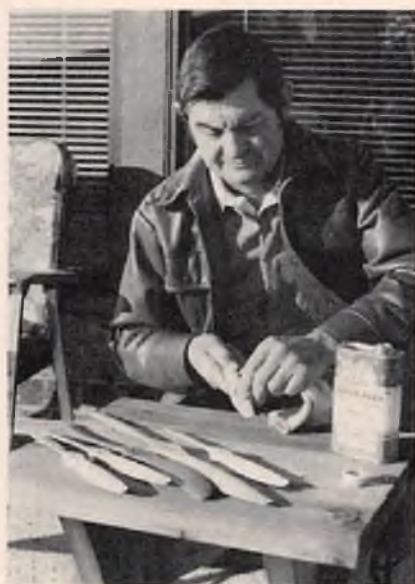
(1) Cleaning finish from prop with a rag and K & B thinner.
