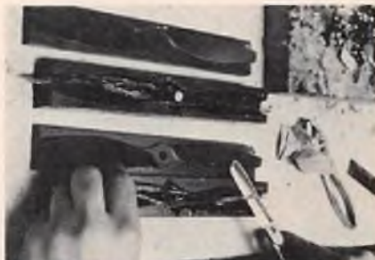
Fiber strands are cut to length and layed in the female half of the mold.
