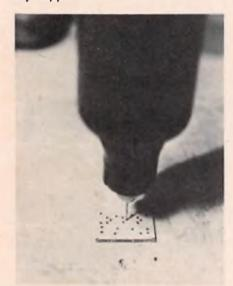
Drill the holes with a #59 drill.
