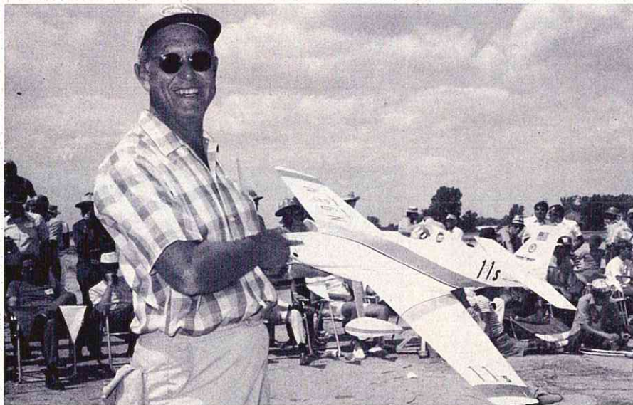
D.C. May had Stegall Minnow, K & B .40 for 17th place. 60% nitro fuel, Kraft radio.
