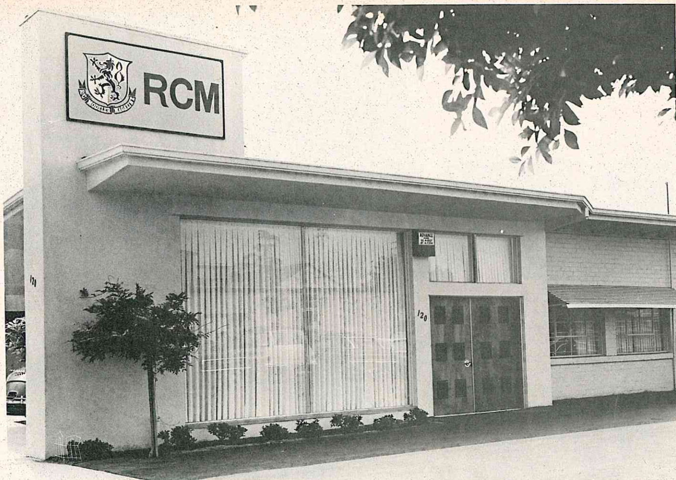
The front portion of RCM's new 6000 square foot home office facility in Sierra Madre, California.
