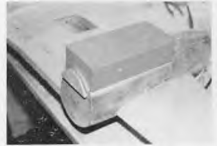
Foam block cemented.
