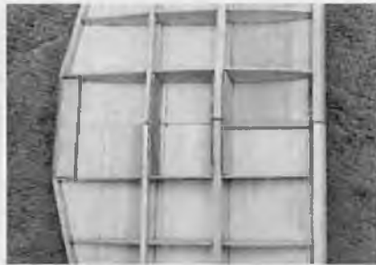
Plywood braces and top sheeting.
