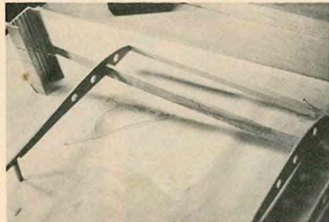
Spar is aligned at tip and held in place. T/E of rib is blocked up to match front spar.
