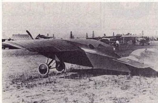
Columnist's next scale project --- the 1920 Pacific C-1 OX5-powered racer, designed by Otto W. Timm. Model will be Quarter Scale from original Timm drawings --- with an Enya 4-cycle .90. Photo courtesy Major Truman "Pappy" Weaver.
