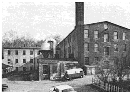
Sterling's present factory — 40,000 sq. feet erected by the "pioneers" in 1886. Walls are 20" thick.
