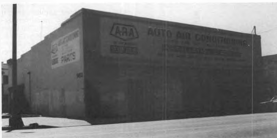
ARA Auto Air Conditioning now occupies the building at 5452 W. Adams St., Los Angeles. The highly regarded Dooling racing engines were built here in the 1940's.
