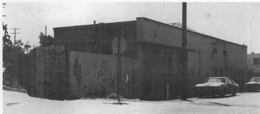
The popular Contestor engine, designed by Dan Bunch, was manufactured at 2636 Humbolt St., Los Angeles. Building is now used by Pacific Packaging Machinery Co.
