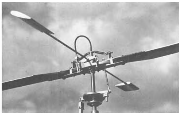
"Scorpion Two" main rotor head, featuring "Bowden Cable" control for collective pitch and Hiller system (cyclic).
