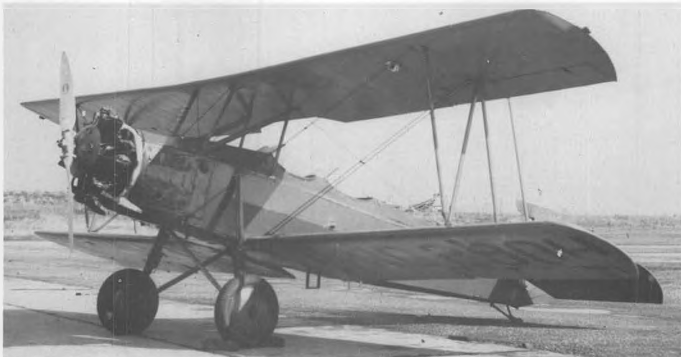
In an effort to improve high speed and rate of climb, Curtiss engineers designed the Fledgling Jr. with 7-1/2 feet chopped off the wings. The Navy also tested the Jr., but performance was no better than the long-wing version. Pete Bowers photo.
