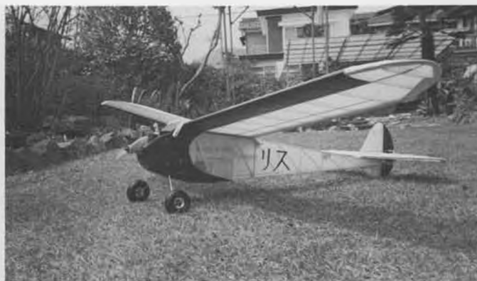
14. Shimpia Yamamura enjoys old timers in Japan with original Japanese designs, this one a 1942 YMK 306 modernized with R/C and an O.S. 20 four-cycle engine.
