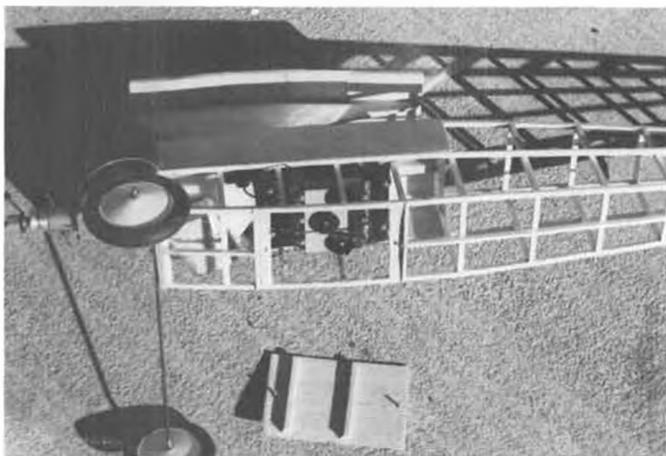
Hatch built into bottom of fuselage provides access to Kraft radio installation. Not bad work for an amateur builder!
